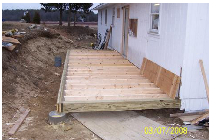
New floor framed out.
