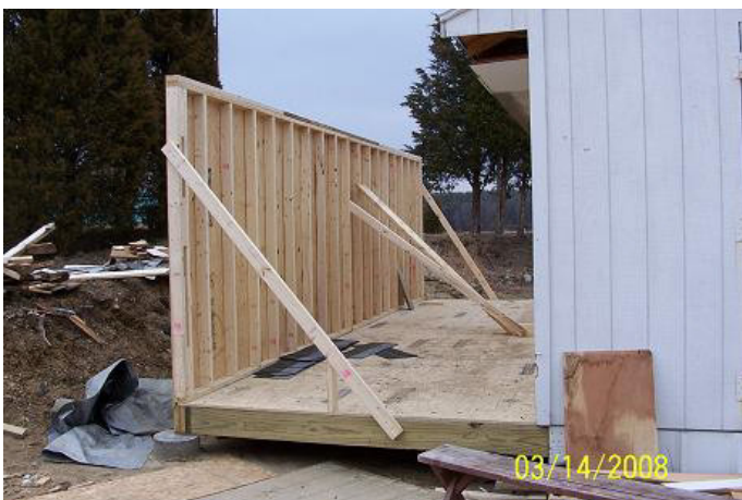
New back wall in place.
