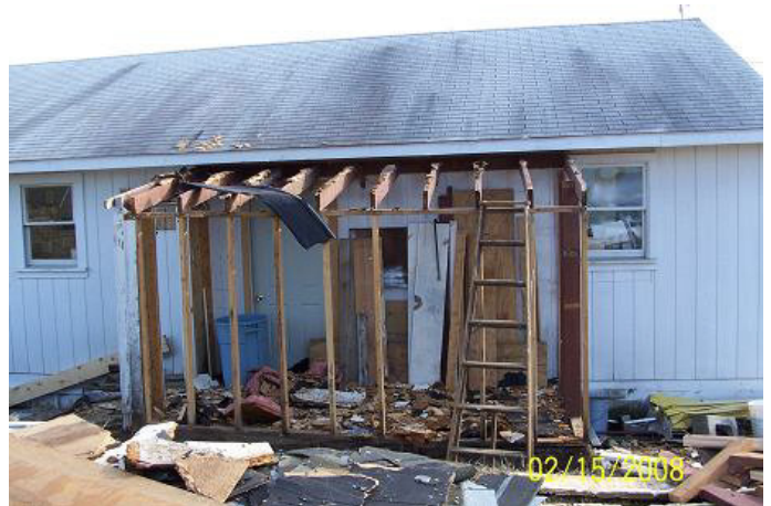
Outer walls torn down.
