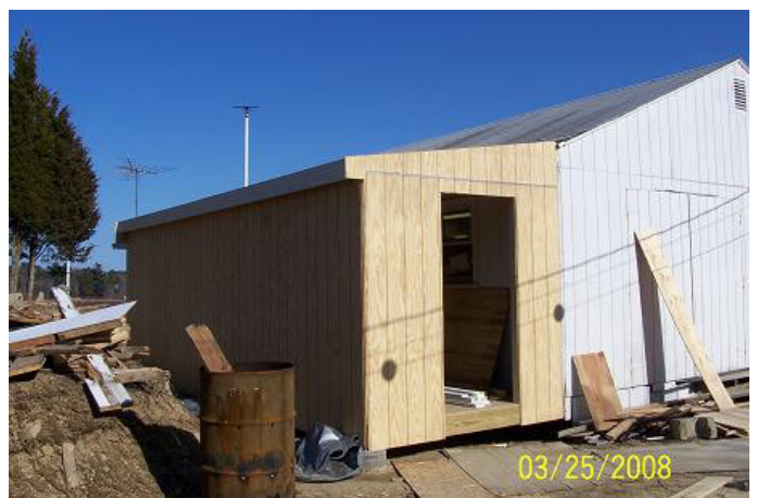
Walls and roof on.
